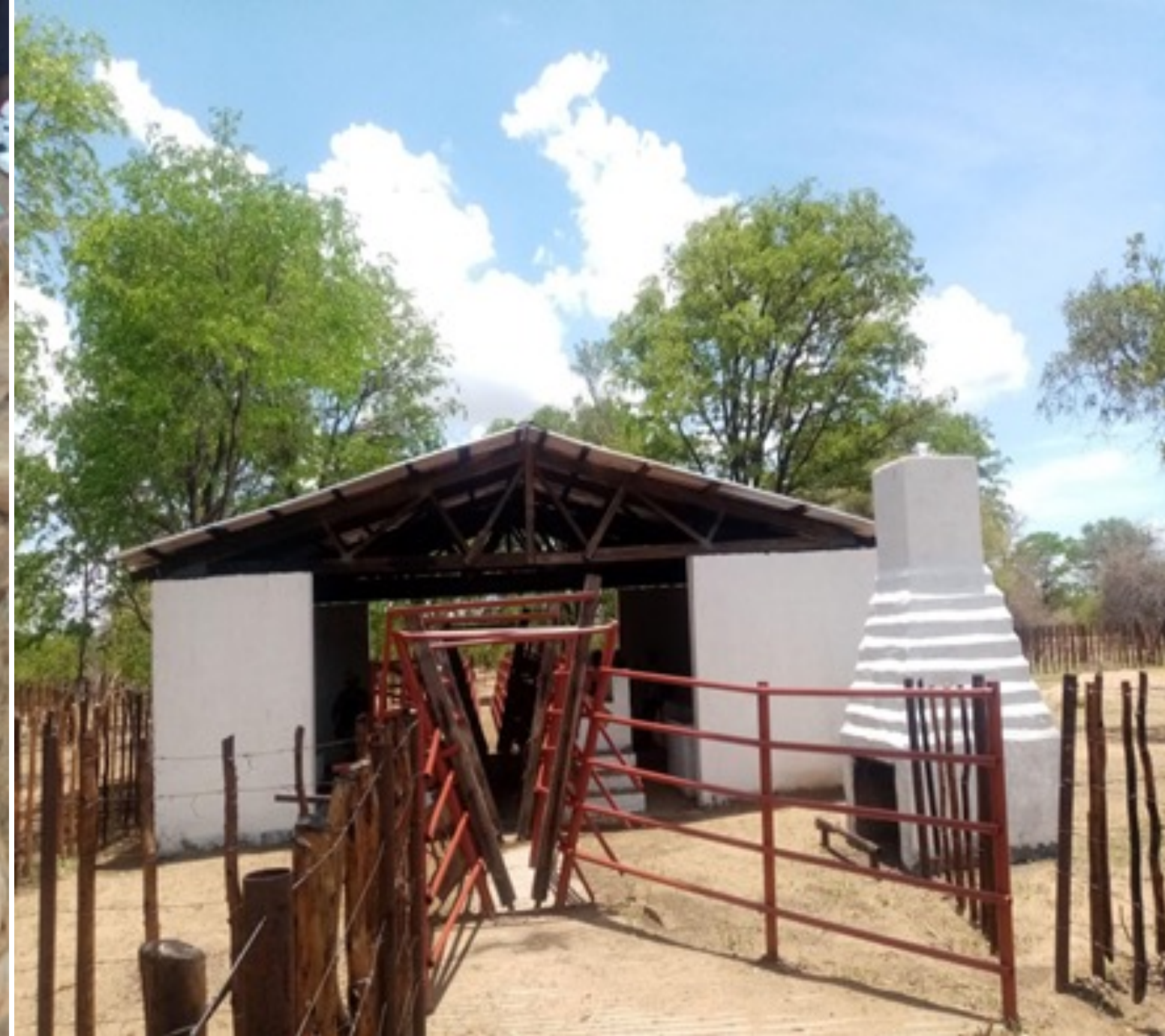
Refurbished cattle sale pens at Jalume, Tsholotsho District
